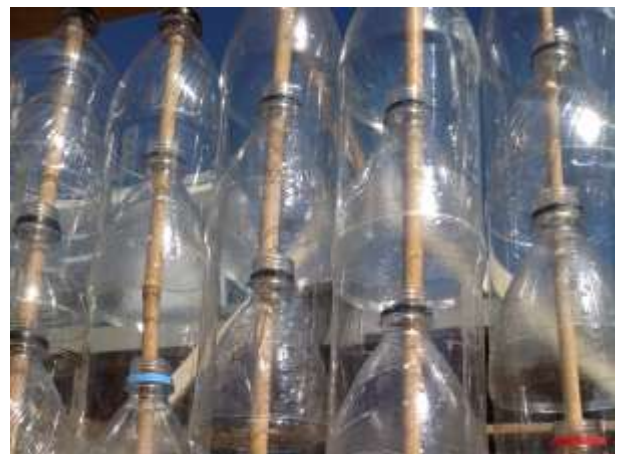
Above: drink bottles are threaded on to garden canes to make the walls. Left: the finished hothouse.
